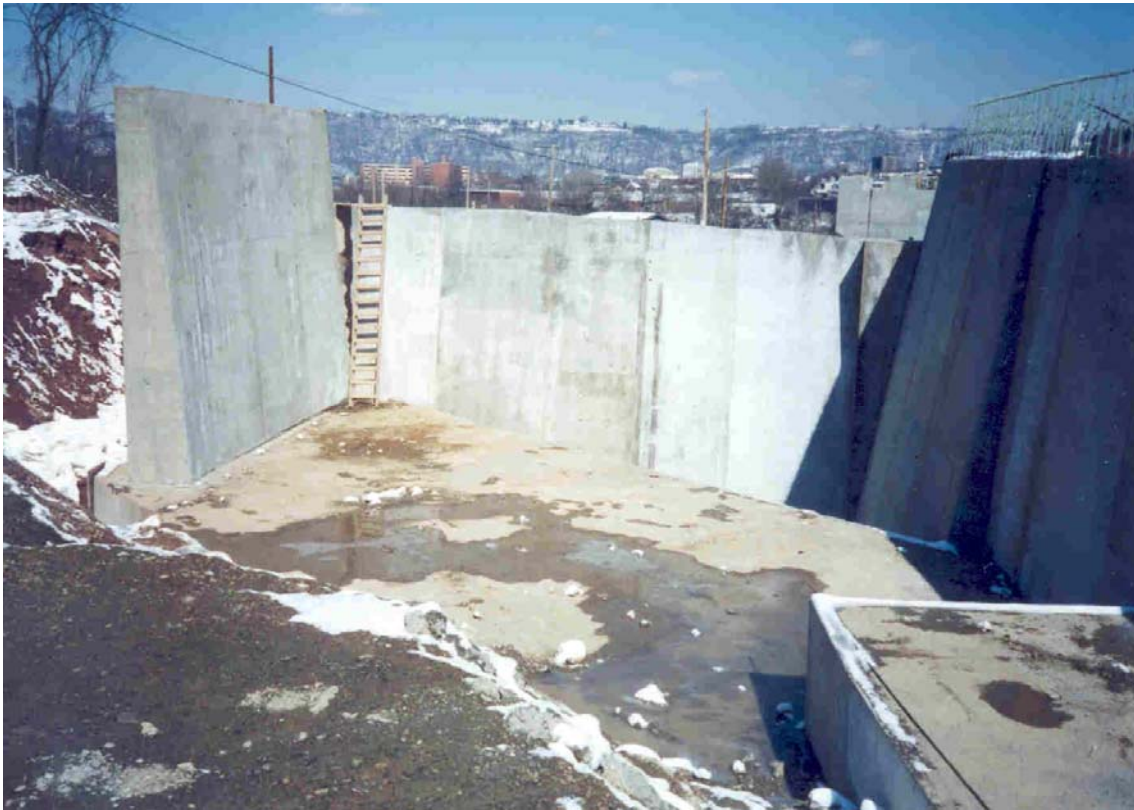
Figure 10-18. CIP abutment with integral wingwalls
