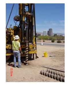
(a) (b) Figure 3-5. (a) Large diameter auger, (b) Small diameter continuous flight auger.
