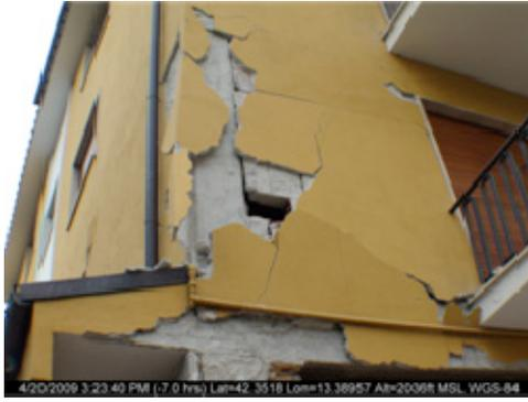
(a) Infill wall-frame separation and corner crushing of the infill wall
