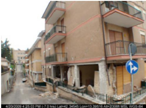
(e) Another building with infill wall failure
