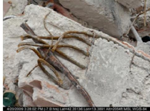
(b) Completely collapsed building with smooth bars and insufficient ties
