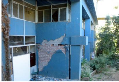
(a) Infill wall damage protecting the frame
