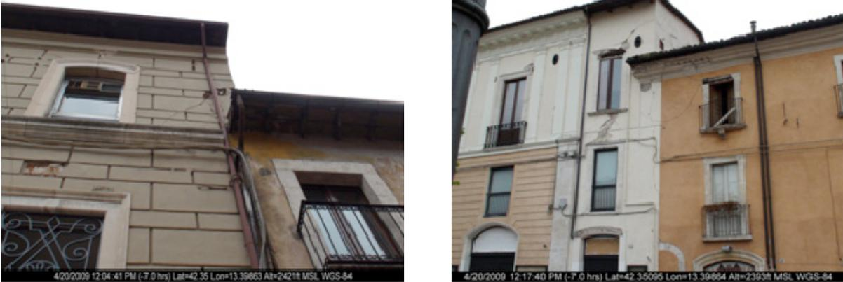
(b) Damage in aggregated buildings as a result of different heights of adjacent buildings
