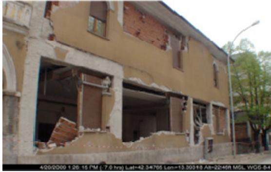
(a) Building with infill wall failure (view 1)
