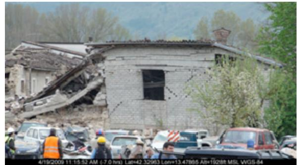
(f) Disintegration of masonry material
