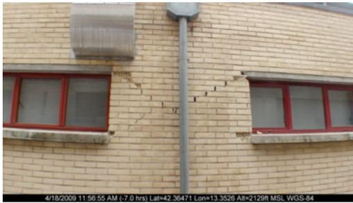
(c) Shear cracks between windows
