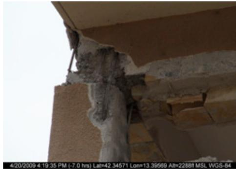
(a) Examples of beam-column joint damage
