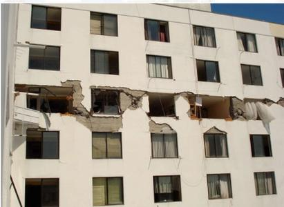
(e) Out-of-plane wall failure at the 9<sup>th</sup> story of a building
