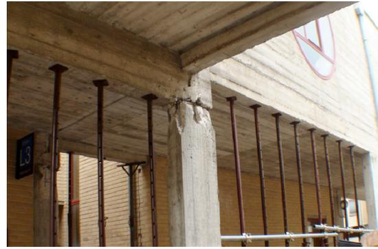
(b) Flexural failure in column
