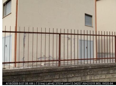
(b) Cracking between RC frame and URM infill
