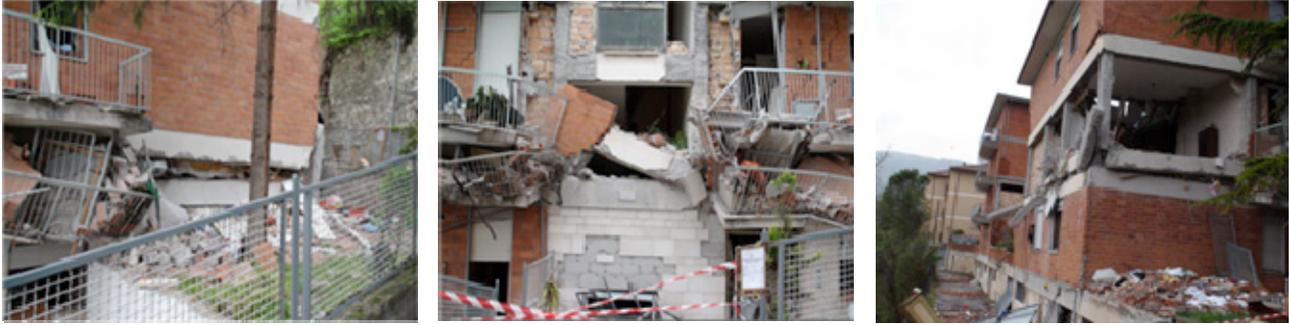
(a) Infill wall failure initiated mid-story collapse
