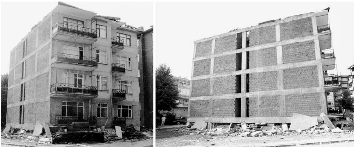
**Fig. 5.1 Building with first two stories collapsed — Kocaeli earthquake**
