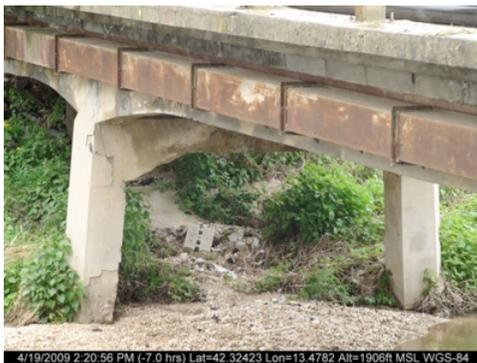
(a) Damage in a RC pier
