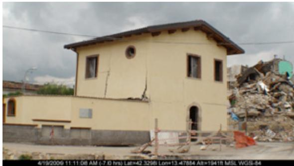
(e) Flexural damage in masonry wall
