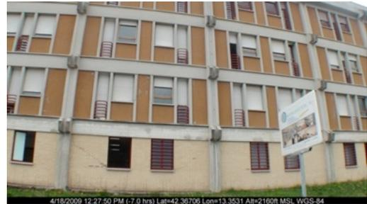
(f) Diagonal crack in first-story infill wall
