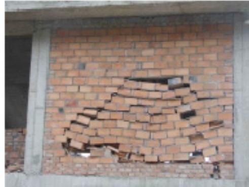
(b) Infill wall shear damage
