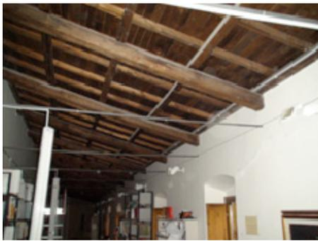
(c) Cross-ties used for out-of-plane restraint
