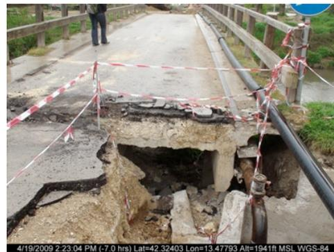
(b) Damage in an abutment due to soil failure
