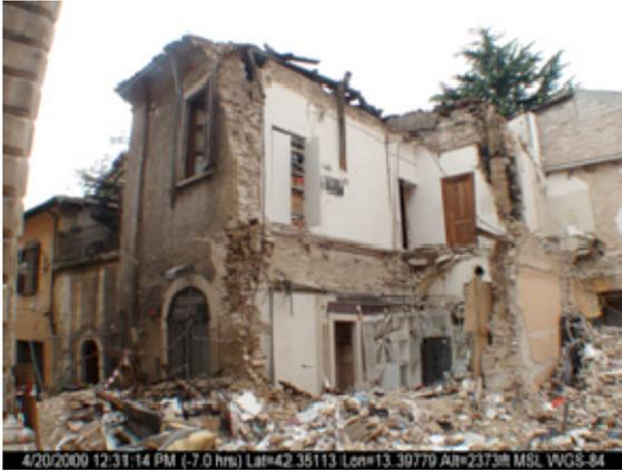
(c) Partial collapse of a building at the edge of aggregated buildings
