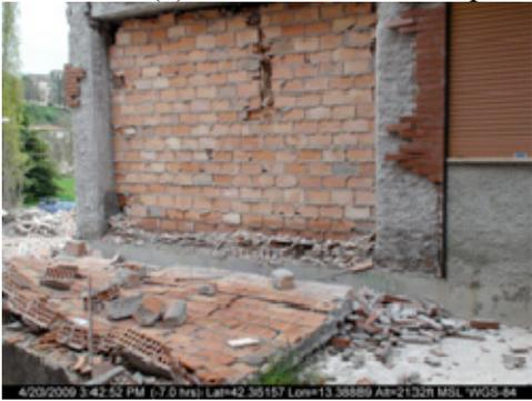
(b) Out-of-plane failure and corner crushing of the infill wall
