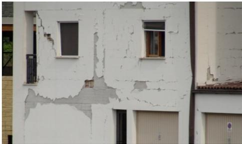
(e) Diagonal crack in infill wall near a window
