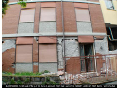
(c) Infill wall-frame separation and diagonal cracking in the infill wall
