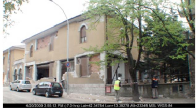
(b) Building with infill wall failure (view 2)
