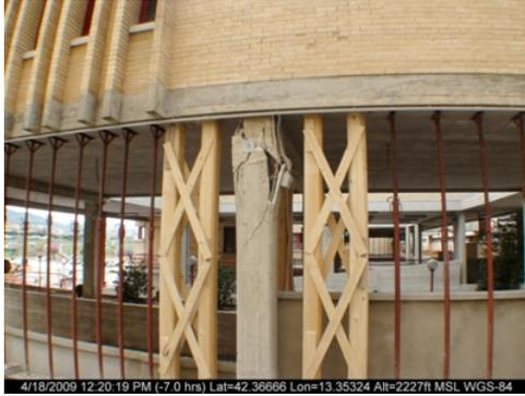
(a) Shear failure in column due to insufficient shear reinforcement
