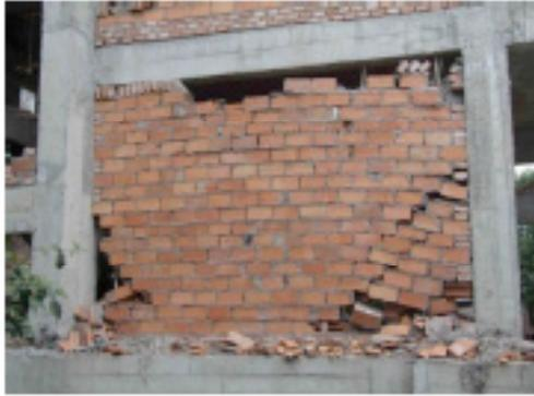
(a) Infill wall compression and shear damage
