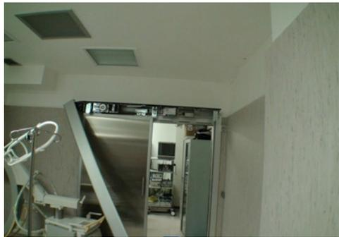
(c) Interior damage of mechanical doors
