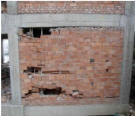
(c) Infill wall compression damage
