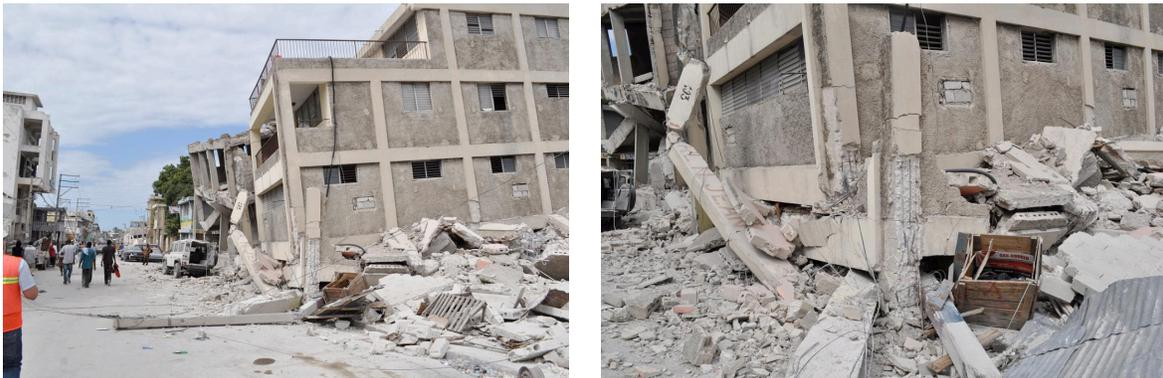
**Fig. 5.2 Building with first story collapsed — Haiti earthquake (photographs by E. Fierro)**
