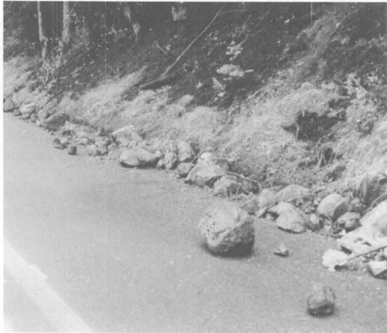
Figure 5.28 Block size used to rate this event.
