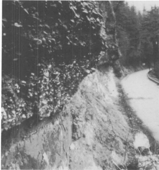
Figure 5.11 The measured sight distance is 330 feet.
