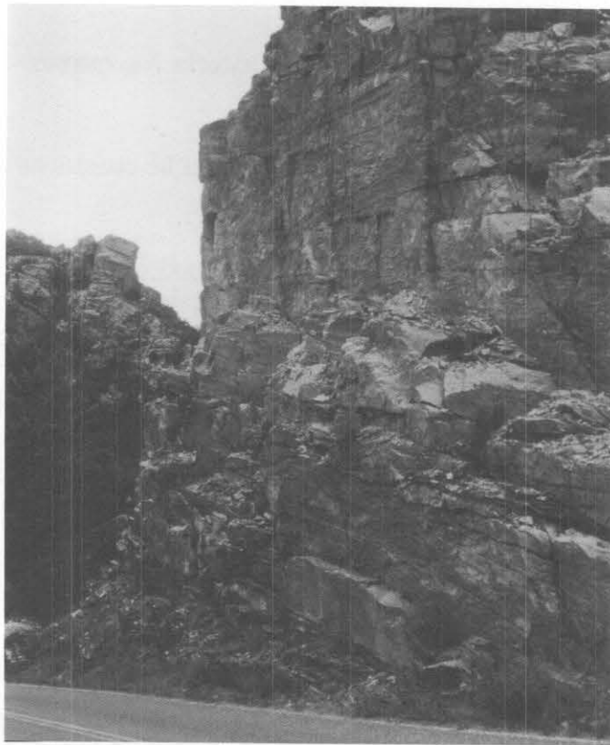
Figure 5.5 The launch feature midway up the slope adds to the ineffectiveness of this narrow roadside ditch.
