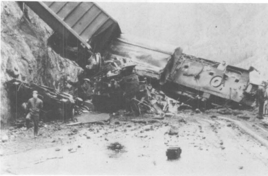
Figure 1.2 Railroad accident caused by a rockfall.
