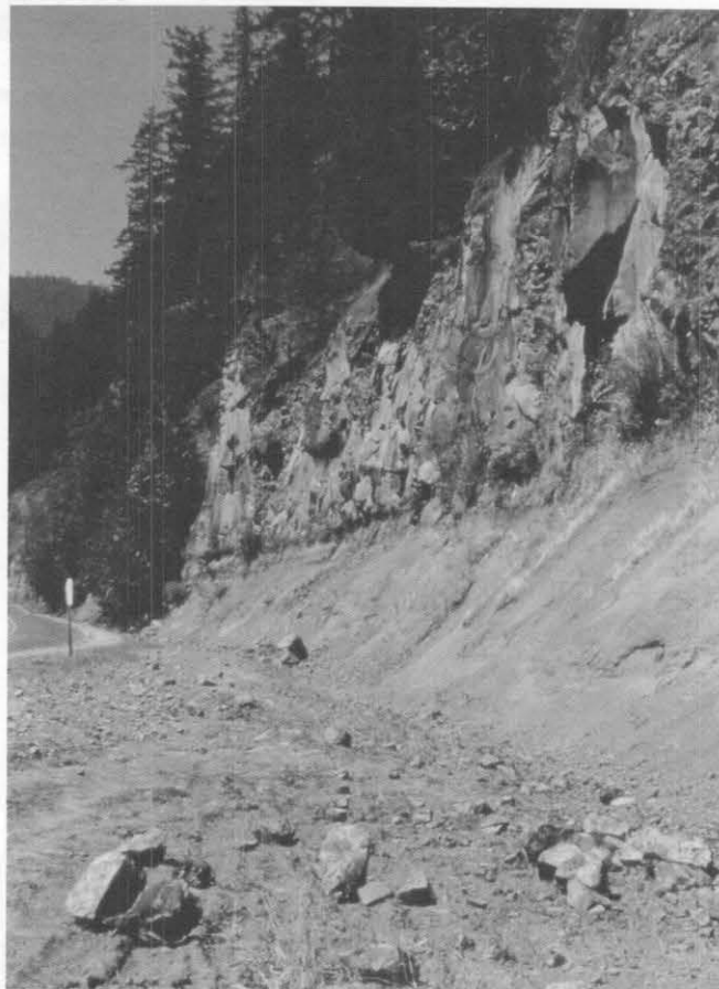
Figure 5.4 The width of this fallout area provides good catchment.
