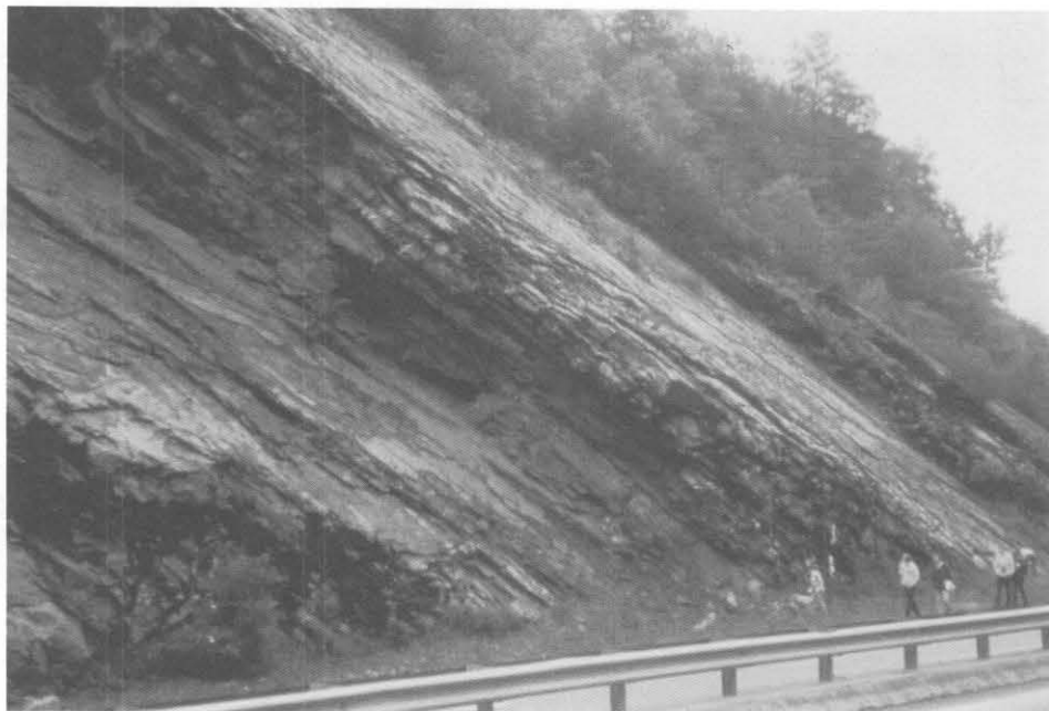
Figure 5.17 Continuous joints with adverse orientation.
