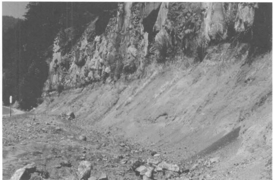
Figure 3.2 "B" rated slope.
