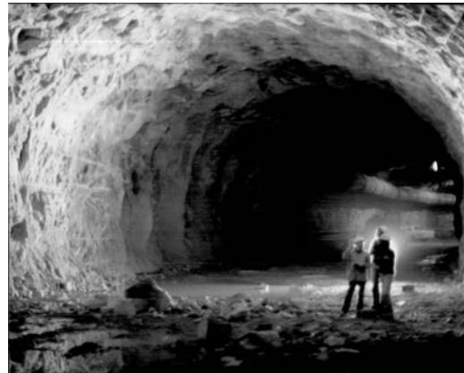
Fig. 13. Top heading for the 12 m span, 18 m high tailrace tunnel for the Rio Grande Pumped Storage Project.
