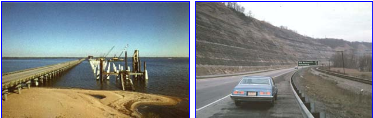
Figure 2-1: New Highway Construction: (a) Pile Bent Bridge in NC and (b) Cut Slope in VA.
