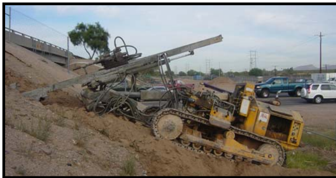
Figure 6. Track rig installing hollow-core soil nails on a slope.
