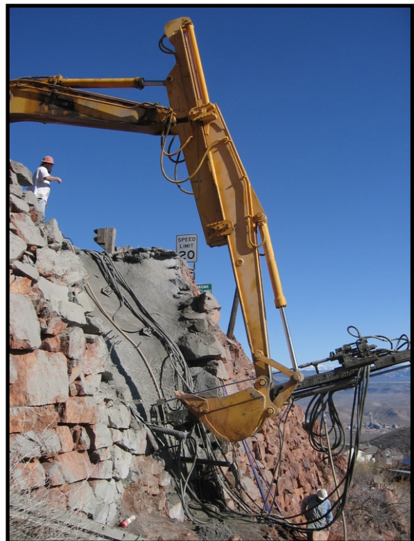
Figure 7. Excavator-mounted drill rig installing hollow-core soil nails to repair a rockery wall in a remote area.
