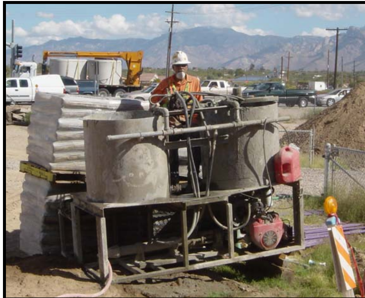
Figure 12. A typical paddle mixer with a holding tank.
