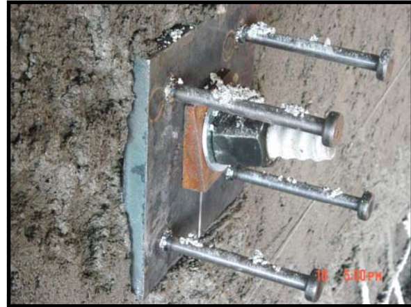
Figure 18. Headed stud bearing plate with a beveled (wedge) washer and a straight hex nut.
