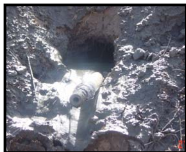
Figure 24. Front view of finished hollow-core soil nail with PVC tube.
