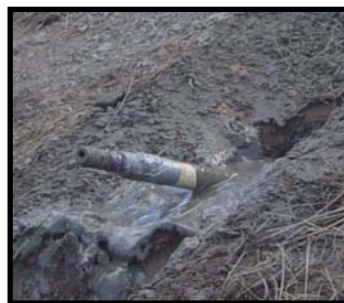
Figure 25. Side view of finished hollow-core soil nail with PVC tube.
