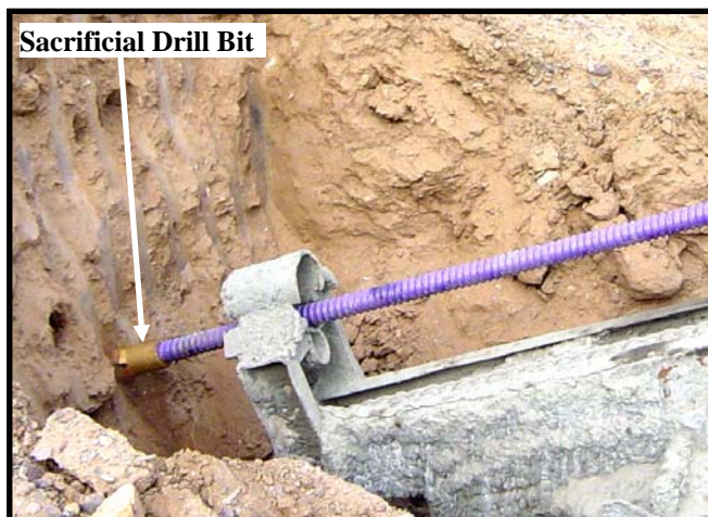
Figure 14. Drill bit attached to a hollow-core soil nail.
