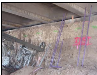
Figure 32. Placing the correct length of hollow-core nail next to the drillhole.
