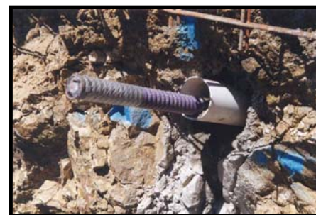
Figure 26. Trimmed PVC tube to expose the hollow-core soil nail for testing.
