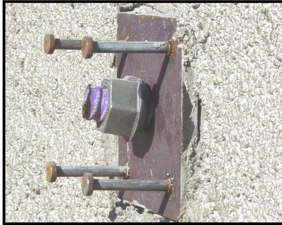
Figure 17. Headed stud bearing plate with a spherical hex nut.
