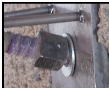
Figure 33. Example of missing beveled (wedge) washer.
