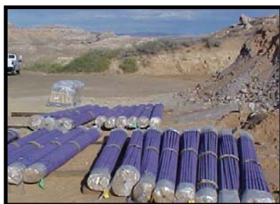
Figure 31. Storage of hollow-core soil nails at site on dunnage.
