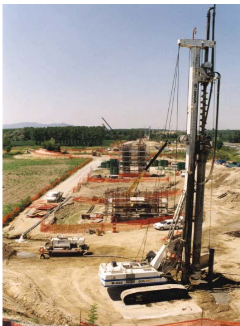
FIGURE 6-12 Drill rig – crawler mounted
