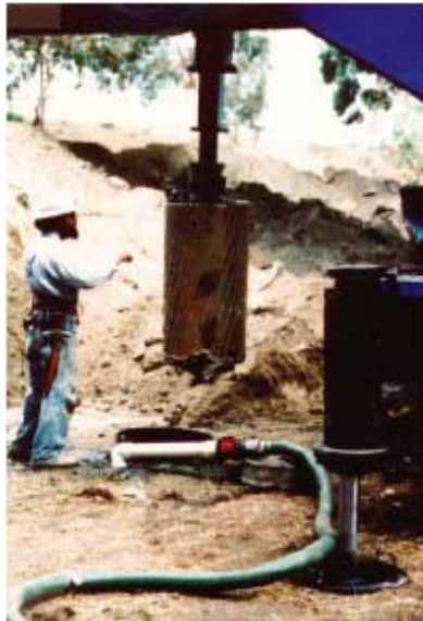
FIGURE 6-4 Drilling bucket
