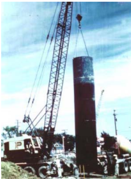
FIGURE 6-11 Steel casing
