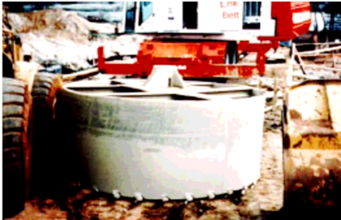
FIGURE 6-6 Core barrel
