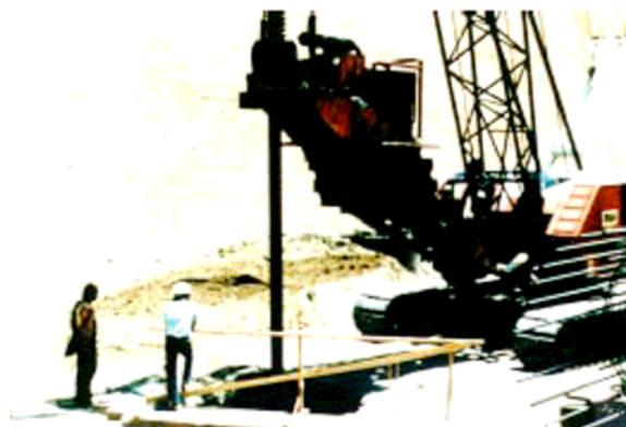
FIGURE 6-14 Drill rig – crane mounted
