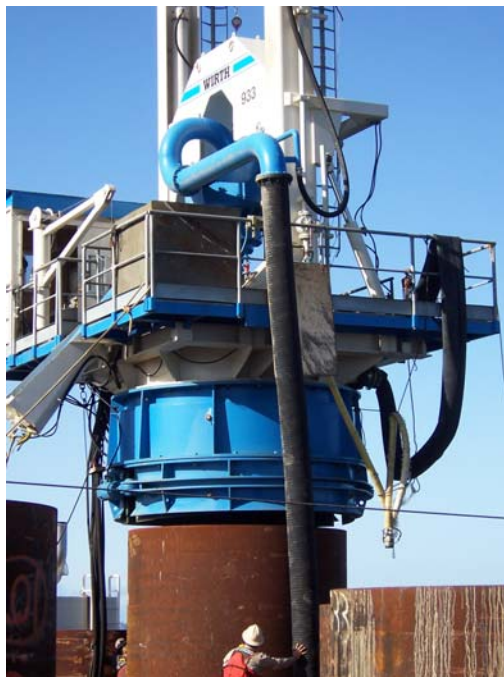
FIGURE 6-10 Reverse circulation drilling equipment
