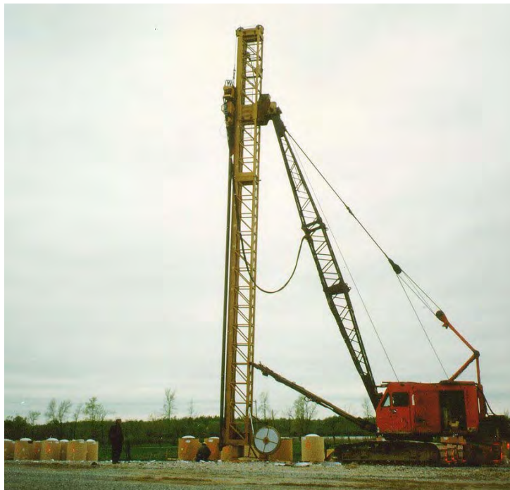
Fig. 4.8 Installation of wick drains type Alidrain (courtesy of J.C. Brodeur, Burcan Industries Ltd.)
