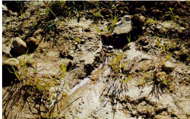
Fig. 4.9 Water discharging from a drain immediately outside the embankment
