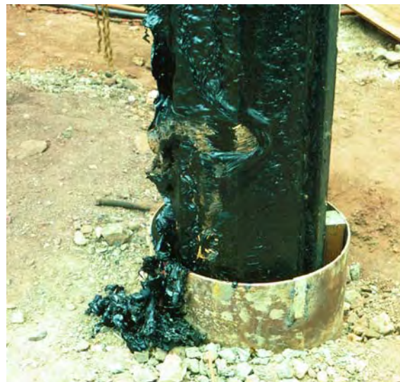
Fig. 7.26 View of a bitumen-coated pile driven through a protective casing. The left side of the pile was the pile underside in storage.
