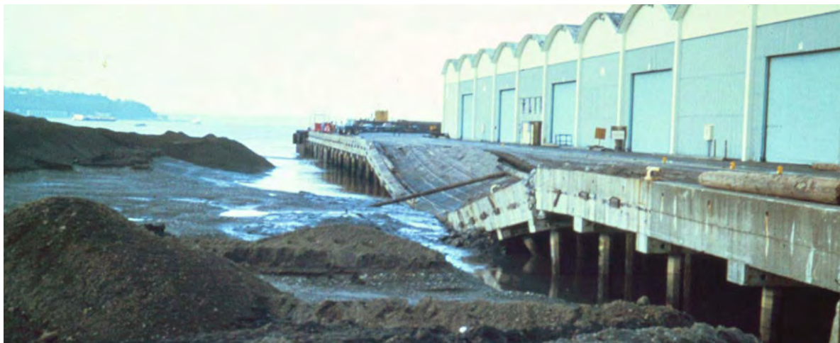
Fig. 7.28 View of the consequence of a hydraulic fill of fine silt flowing against 24-inch piles
