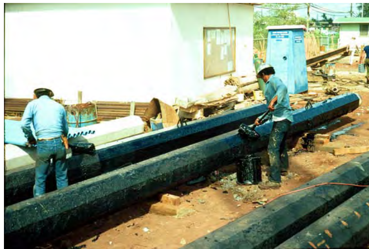
Fig. 7.26 View of work under way to apply a bitumen coat to a concrete pile.
